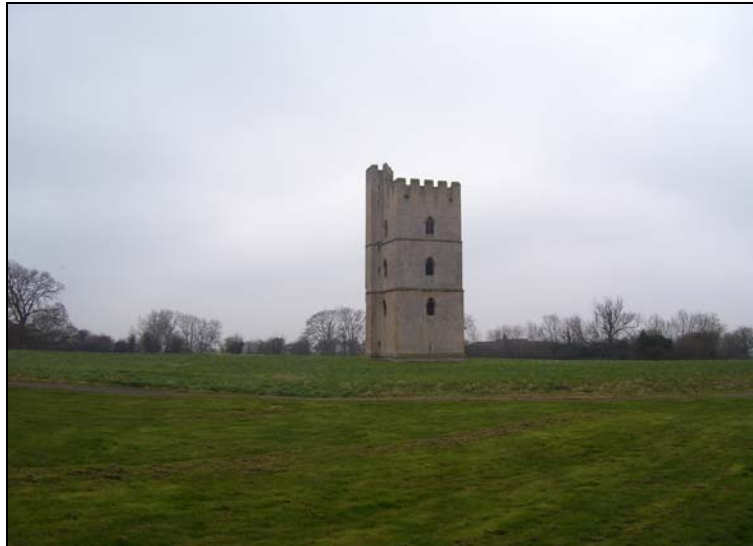
Kyme Tower to the west of South Kyme village
